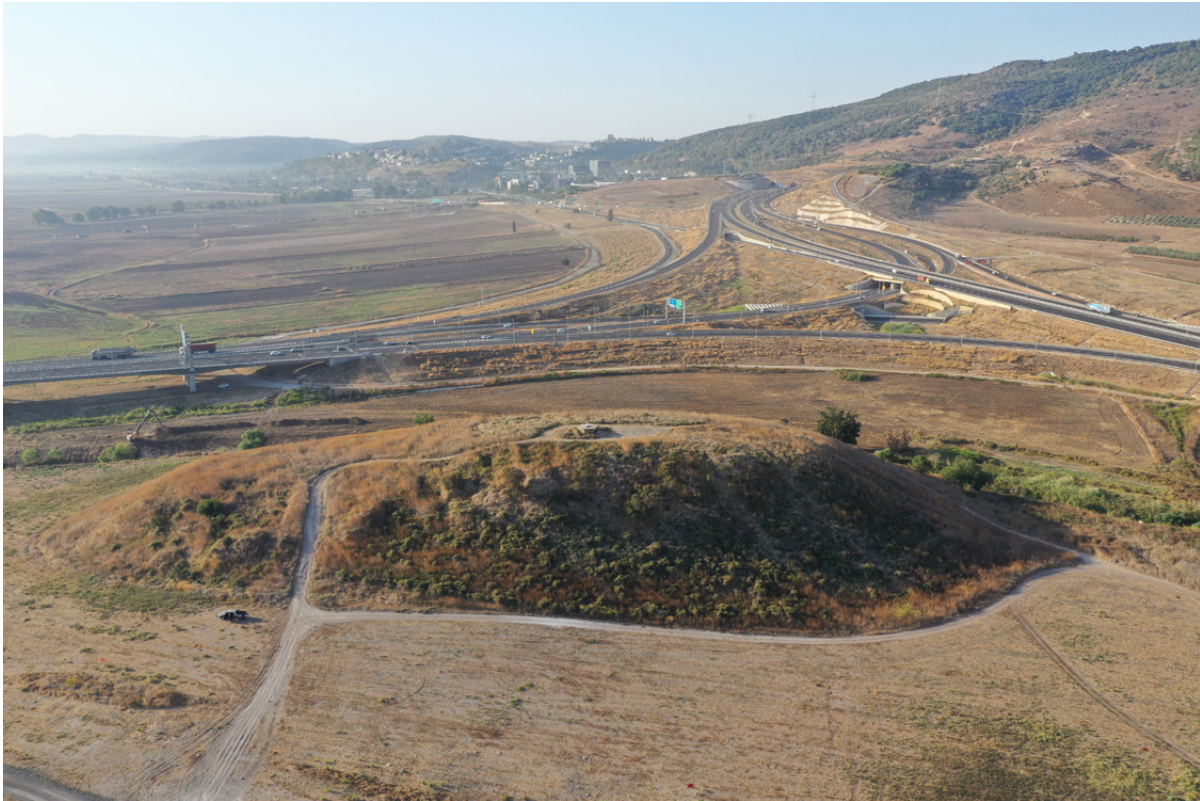
Fig. 1.6. Aerial view of Qashish region after the completion of infrastructure works, looking south toward Yoqne'am. Courtesy of the JVRP.
