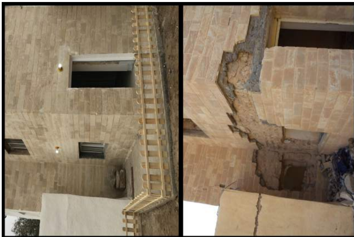
Fig. B1.6: The façade of the southeastern block of the excavation house, before and after restoration. Photos by Akam Omar Ahmed Al-Qaradaghi.
