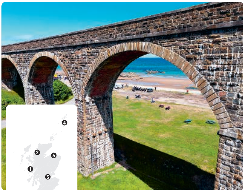
Cullen Viaduct (p. 221)
