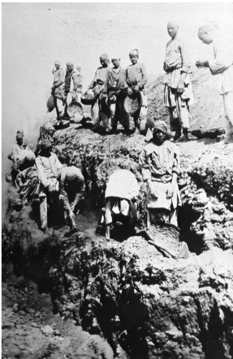
Figure 1.6. Deep-level excavation, probably in 1903. Photo from glass negative in the Papyrology Rooms, Sackler Library, Oxford.
