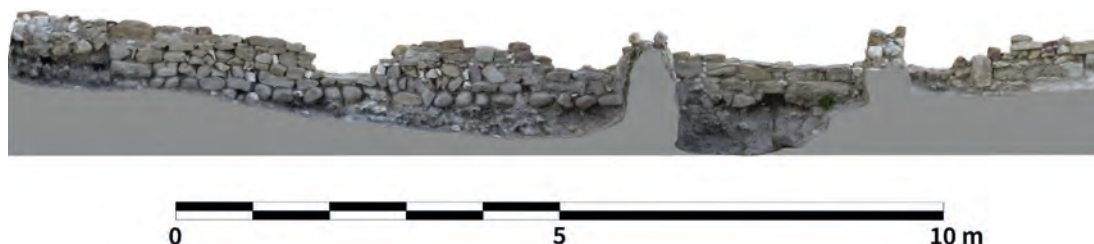
Fig. 20. Wall W16 (from the north).
